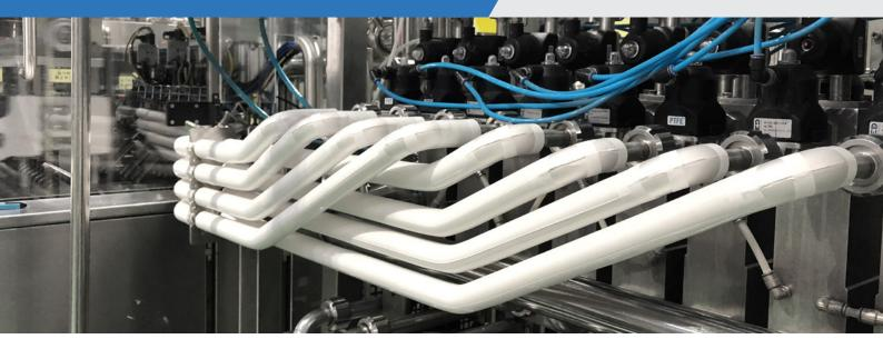
T-FIT® Hygiene insulation is made from Zotefoams' ZOTEK® F43HT PVDF closed cell foam, a material which has numerous benefits when it comes to insulation, especially within food manufacturing environments.
