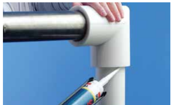
2.6 Adhesive is applied to the elbow joint and secured with tape.
