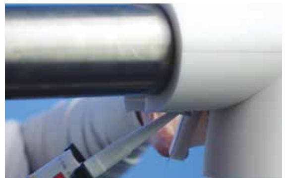
2.6 Adhesive is applied to the elbow joint and secured with tape.
