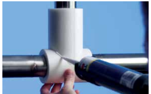
5.7 Apply sealant to the joint between the two parts.
