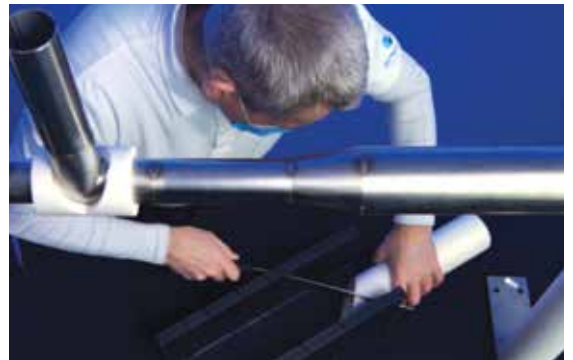
5.5 Ease the straight cut surfaces and tips with a sharp knife.
