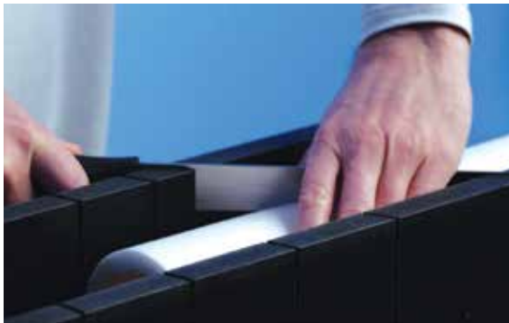
2.1 Using a sharp knife and mitre block, cut the Hygiene tube to length as required.
