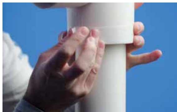
2.7 The elbow fitting is taped and sealed to the adjoining insulation.
