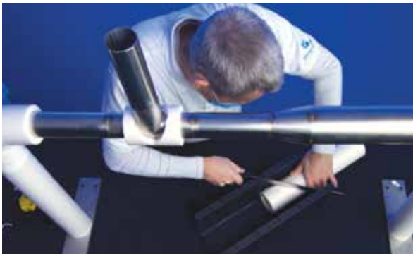
5.4 Taking T-FIT Hygiene straight insulation appropriate to the branch, make two 45° angle cuts to one end.
