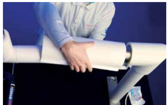
4.4 Install the second prepared T-FIT Hygiene tube.
