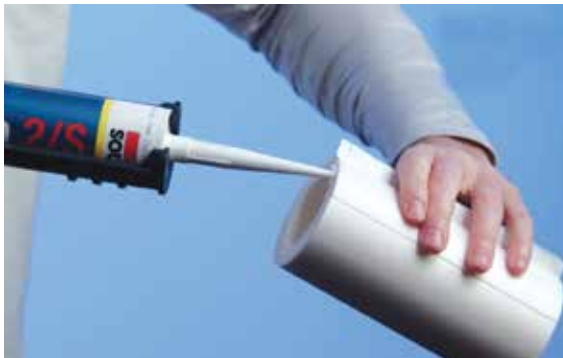
4.1 Carefully apply sealant to the longitudinal joint and the end of the first insulation tube, preparing the butt joint to the next item of insulation. In this example the 38mm / 1.5" tube.
