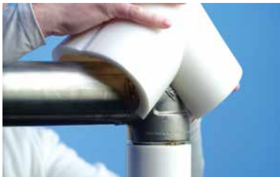
2.5 Image shows installing around the pipework elbow.
