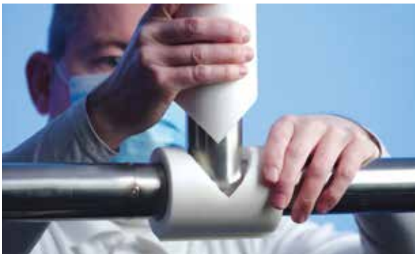
5.6 Assemble the two parts to make up the tee insulation.
