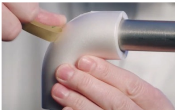
2.3 The fitting is secured with tape cut down to 12.7mm width, applied around the throat of the elbow.
