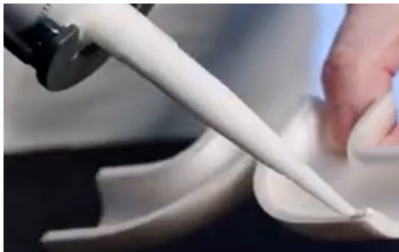
2.1 Apply sealant to the outer edge of the fittings, close up the elbow and leave for ~6 hours for the sealant to cure.
