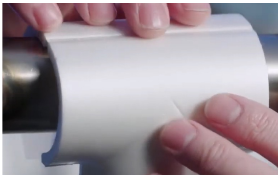
5.3 Install the prepared tee fitting.
