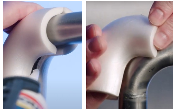
2.2 After the sealant has cured the fitting is installed around the elbow, and sealant applied to the internal edges.
