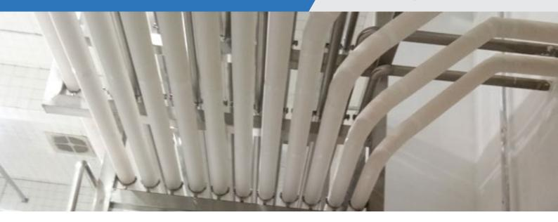
T-FIT® Hygiene insulation is developed from Zotefoams' ZOTEK® F 43 HT PVDF closed cell foam, a material which has numerous benefits when it comes to insulation, especially within food and beverage, dairy and other aseptic, sterile environments.
