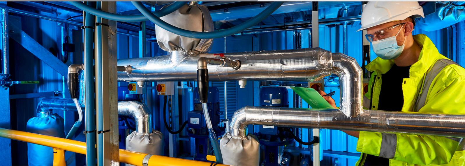
Through internal testing, T-FIT® insulation materials have been shown to provide protection against contact burn injuries from heated surfaces. This document provides a brief summary of the testing and results.
